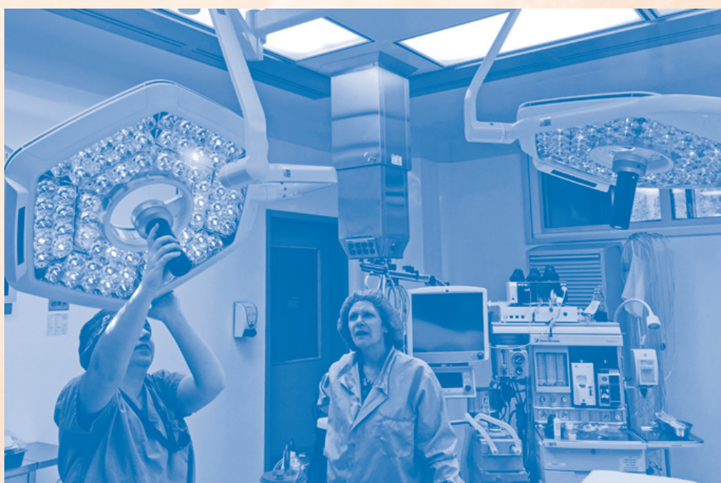
As part of the 'tie-in' process of attaching the new building with the existing hospital, current operating rooms received new upgrades. These energy-efficient, state of the art LED overhead lights (pictured) were installed in both operating rooms to provide better lighting for staff during surgical procedures.
