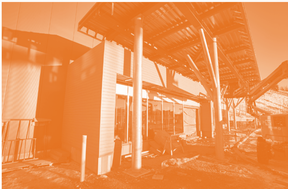
The new emergency entrance is finished using natural-like materials and elements that will be found throughout the new building. Once the canopy is finished, it will look similar to the bottom of a canoe.
